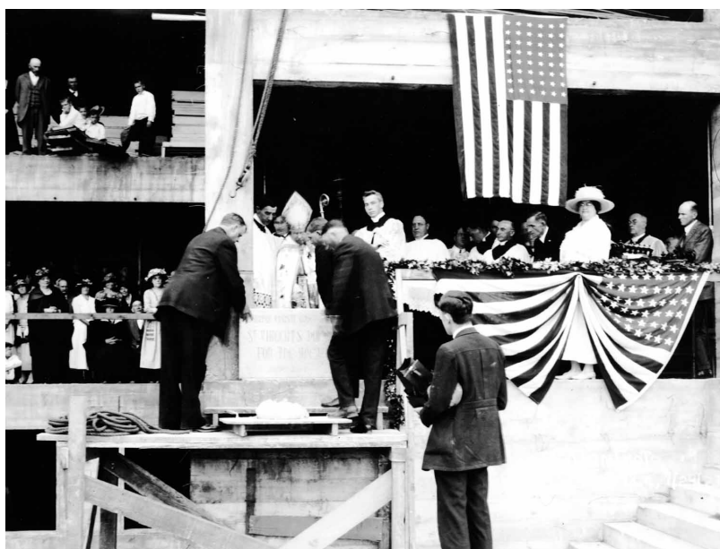
Cornerstone installation at St. Vincent Home for the Aged, now Providence Mount St. Vincent, in West Seattle, July 29, 1923
