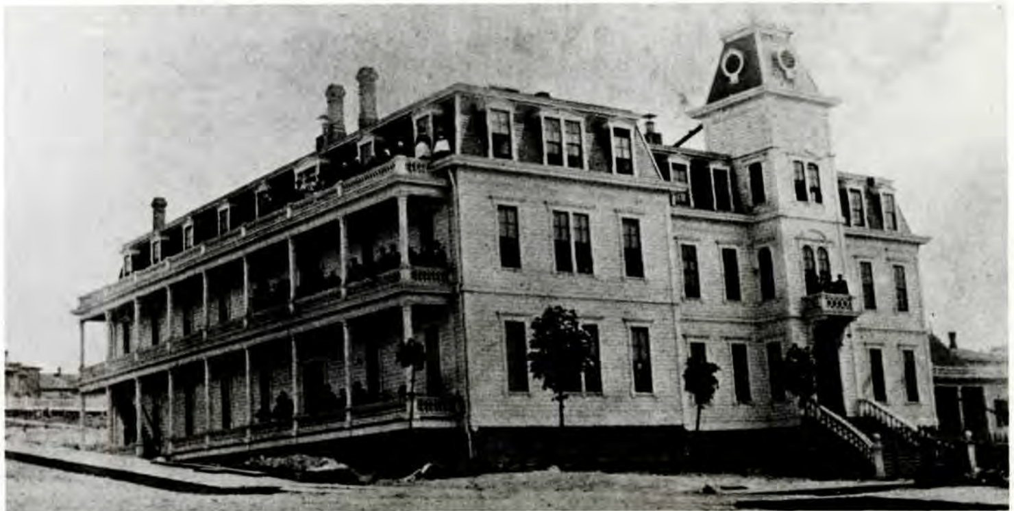
Overcrowded conditions led Mother Joseph to design a new hospital building at Fifth and Spring.
