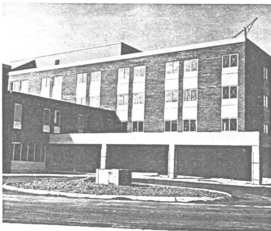
COLUMBUS' NEW HOME. That has double meaning. True the building is the new Columbus Hospital with the outpatient entrance featured. But in the foreground the wooden box shows where the statue of Columbus will be come 1977.
